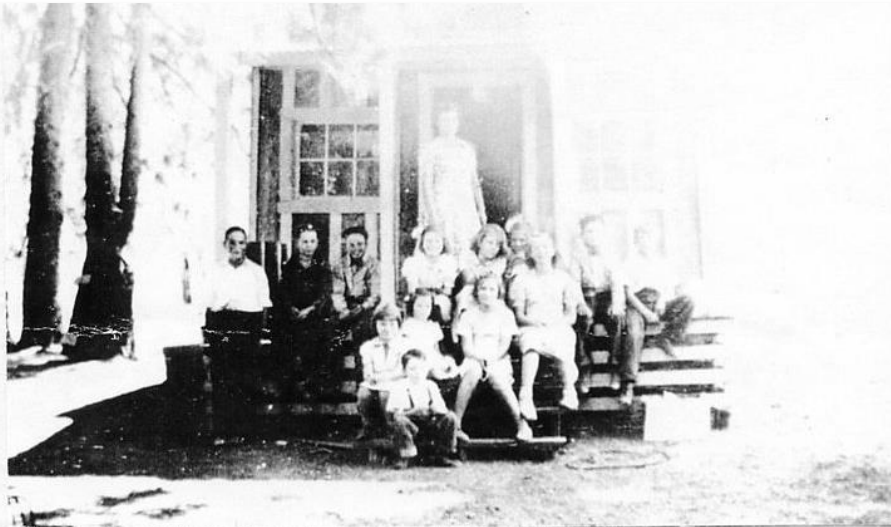
GRASS VALLEY SCHOOL - 1939 looking eastward toward west end of remodeled schoolhouse
